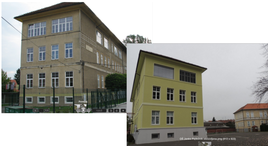
One of the 24 renovated public buildings in the municipality Maribor (primary school)
